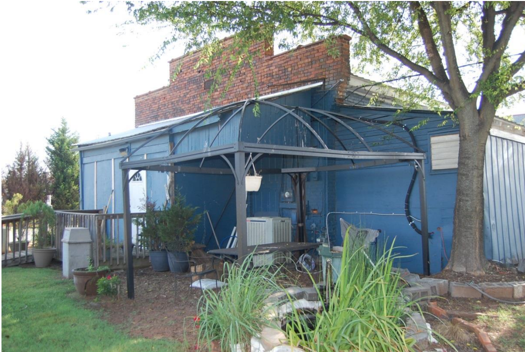
Hayes-Byrum Store, Rear (West) Elevation, Looking Northeast.
