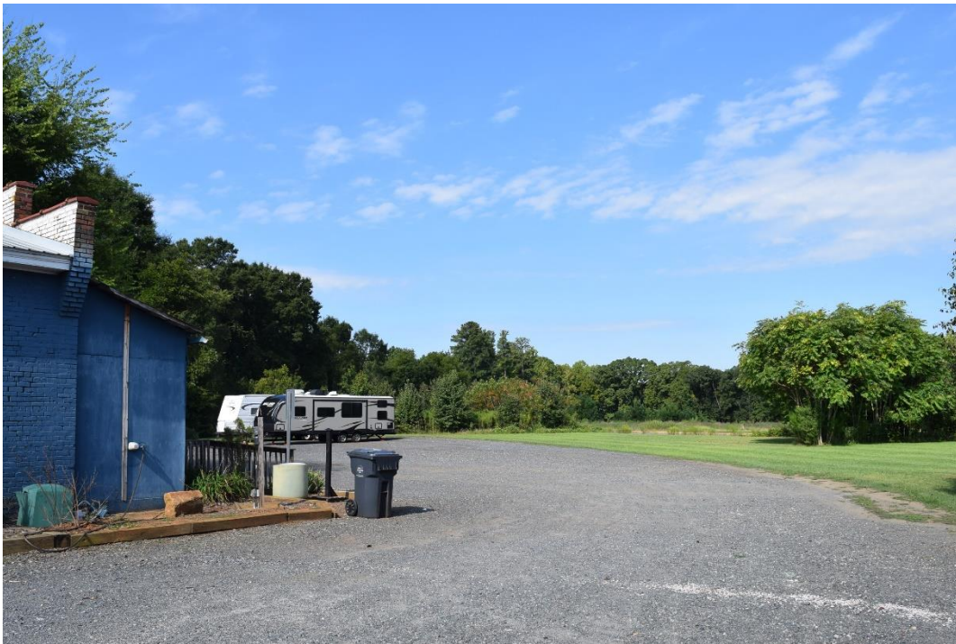
Hayes-Byrum Store, Rear Lot, Looking Southwest.
