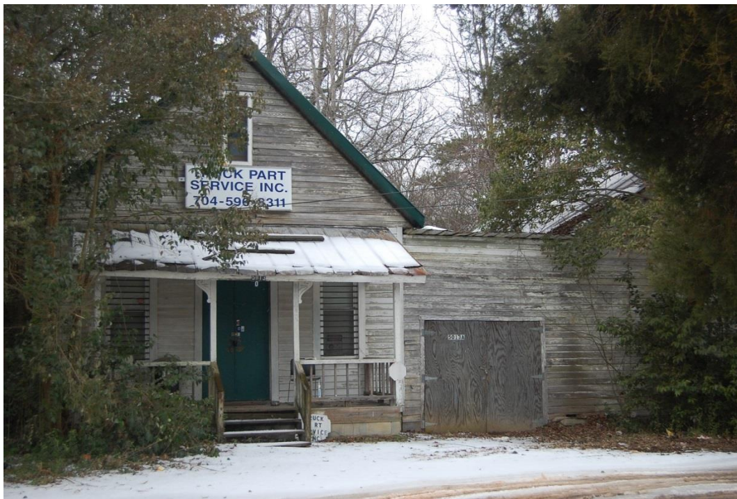
P.T. Christenbury Store, 1909, 5013 Statesville Road, Charlotte. Demolished 2018. (2015 Photograph by Mattson, Alexander and Associates, Inc.)
