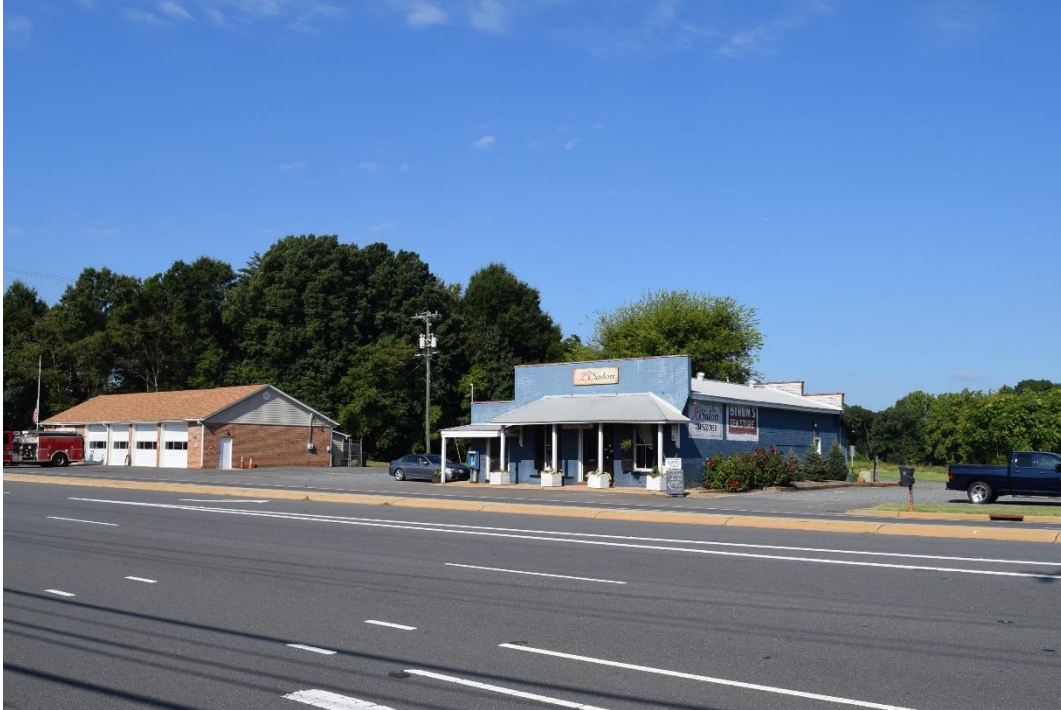
Shopton Historic District, Hayes-Byrum Store and Steele Creek Volunteer Fire Department, Looking Southwest.
