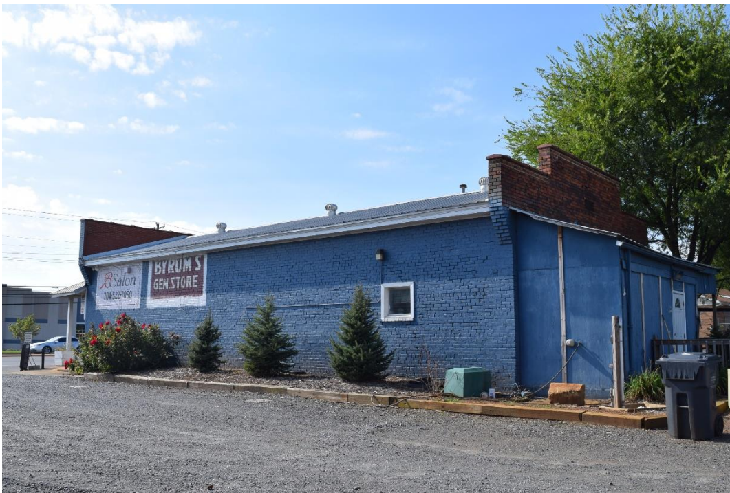
Hayes-Byrum Store, Side (North) and Rear (West) Elevations, Looking Southeast.
